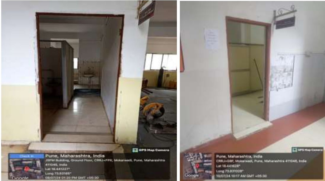
Figure 2: Accessible Gents and Ladies Toilets
