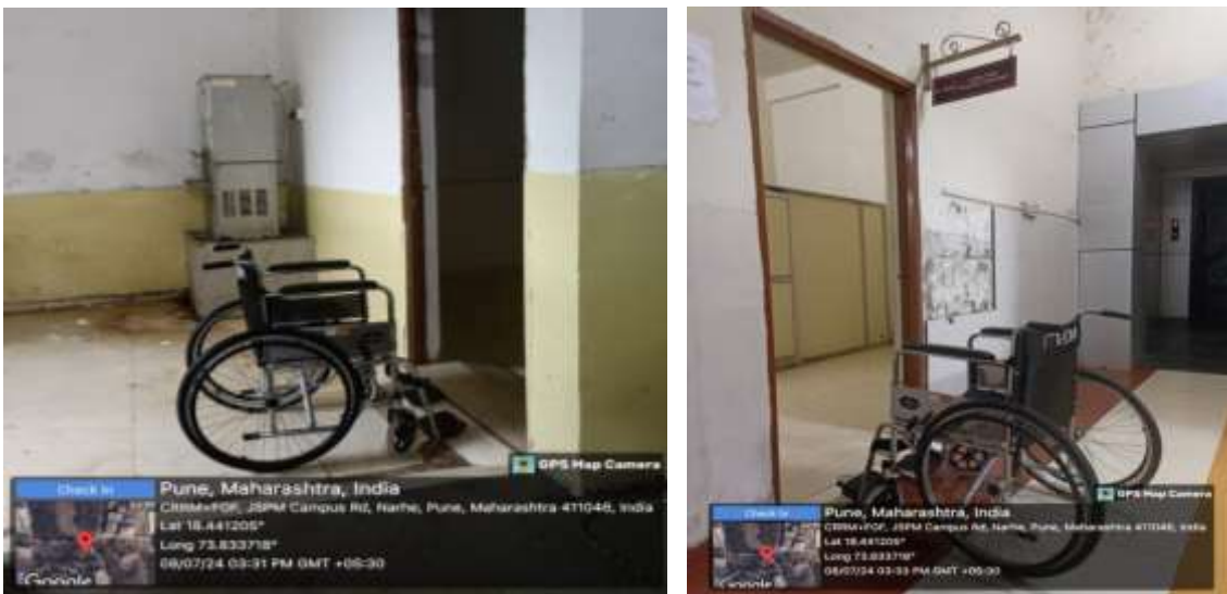
Figure 3: Wheel chair facility
