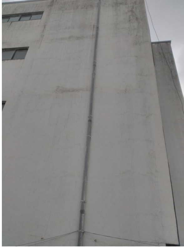
Fig. 1 Photograph of rain water harvesting structure
